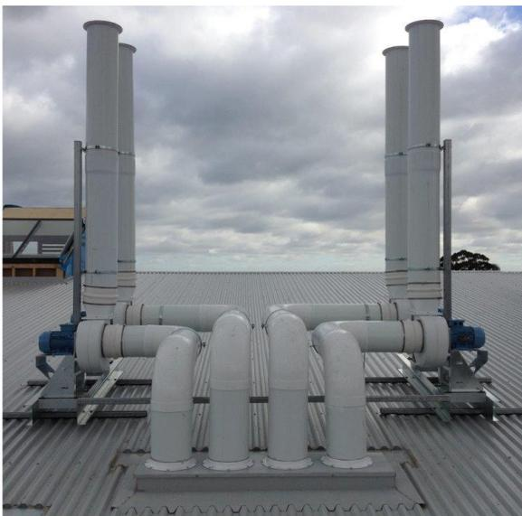
The Laboratory Systems Group range of polyfans are specifically engineered to suit high volume ventilation applications. Constructed from premium quality materials, the VSB-series polyfan range incorporate a highly corrosive-resistant fully metal-free casing with a high efficiency fully balanced impellor.
