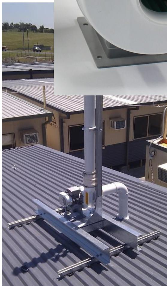
The Laboratory Systems Group range of polyfans are specifically engineered to suit high volume ventilation applications. Constructed from premium quality materials, the VSB-series polyfan range incorporate a highly corrosive-resistant fully metal-free casing with a high efficiency fully balanced impellor.
